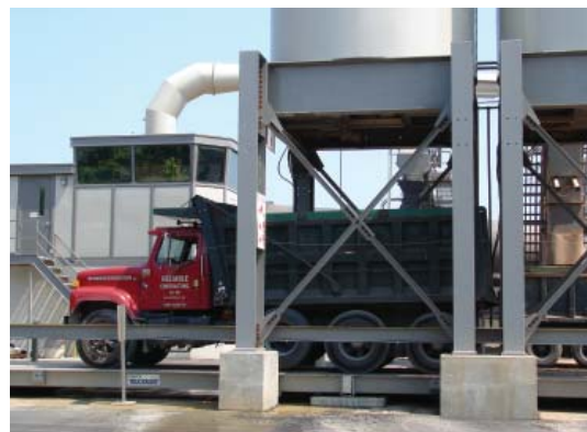
The new three-silo asphalt plant required a longer truck scale.
