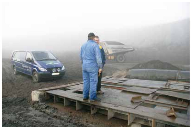
A service engineer of METTLER TOLEDO is upgrading a truck scales with POWERCELL® in Kiruna, Sweden
