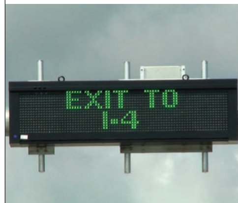
Variable Message Sign (VMS) used to automatically or manually direct driver (i.e. STOP, EXIT, PULL FORWARD, BACK UP, PARK)
