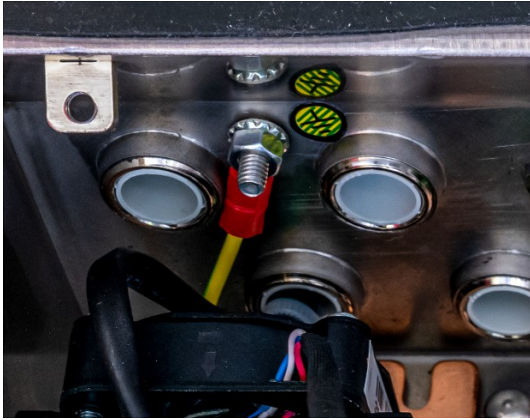
Figure 35: Grounding Bolt, Harsh Environment Enclosure
