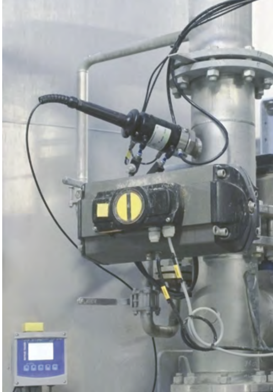
Figure 2: pH measurement point in the process. The sensor is installed with a pneumatic InTrac housing in the pipeline, so no bypass lines are required.
