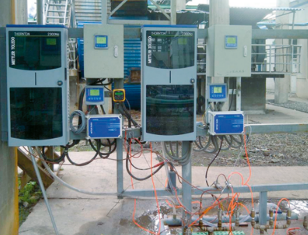
METTLER TOLEDO condensate-quality monitoring systems, including 2300Na Sodium Analyzers, at Jiahua Energy.
