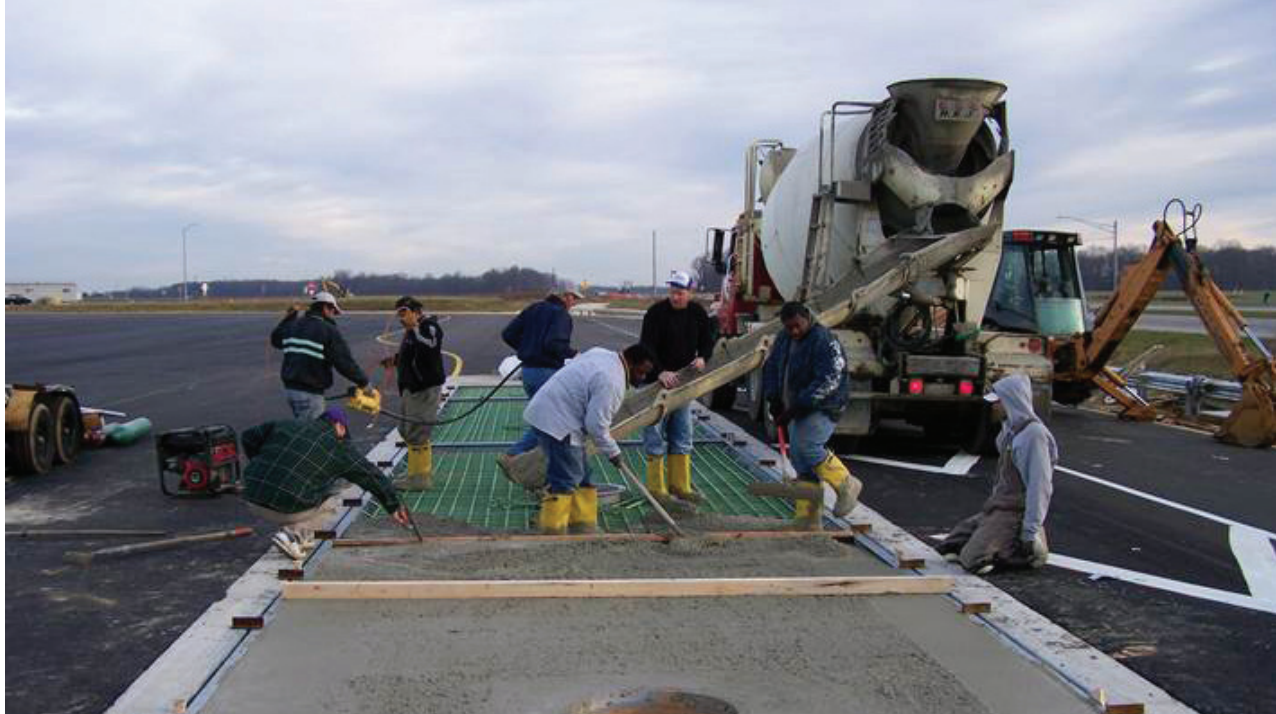
Concrete is poured into the deck of a concrete weighbridge at installation
