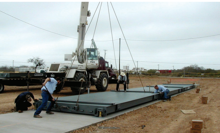
A steel deck weighbridge is installed
