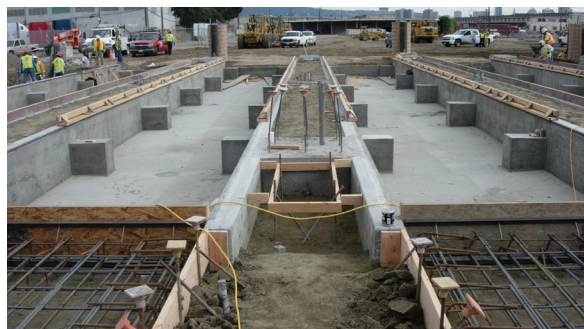
Foundation preparation can take place prior to the scale components arriving on site
