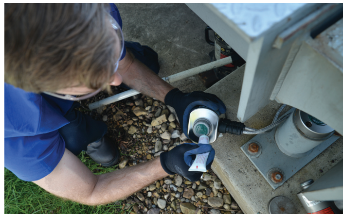
Some areas, such as load cell mating surfaces, require periodic lubrication
