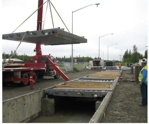
A pit-style scale is placed in an excavated foundation, flush with the ground
