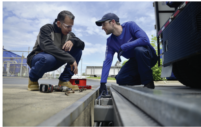
Inspect the scale checking or suspension system to ensure it is adjusted properly
