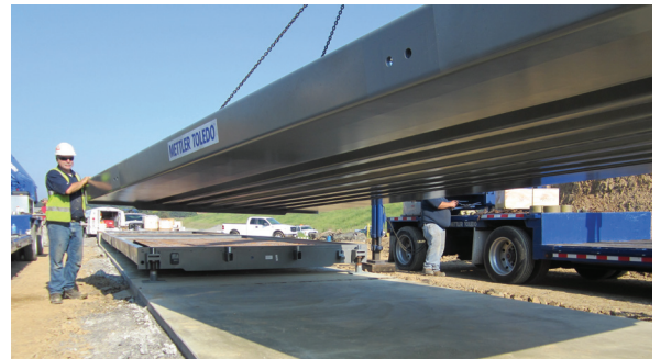
The weighbridge modules are placed into the foundation
