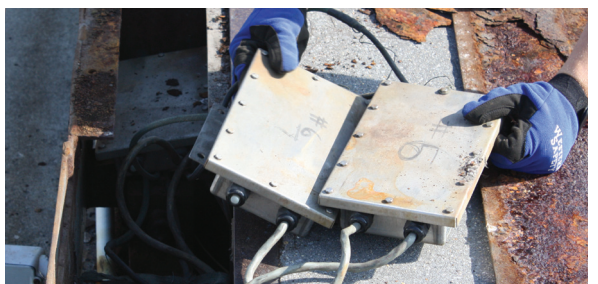
Junction boxes contain circuit boards and many manual wire connections. They are the main cause of truck scale downtime because they are difficult to seal against moisture.
