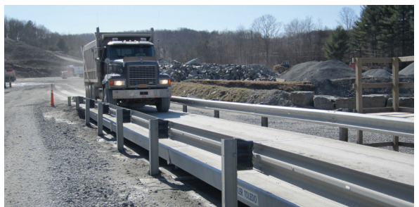
These stand-alone guiderrails are planted in the ground alongside the scale to offer added strength and prevent trucks from driving off the side of the scale
