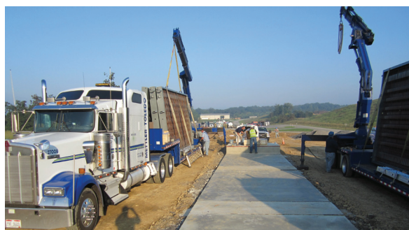
Specially designed delivery trucks are able to transport the weighbridge modules upright
