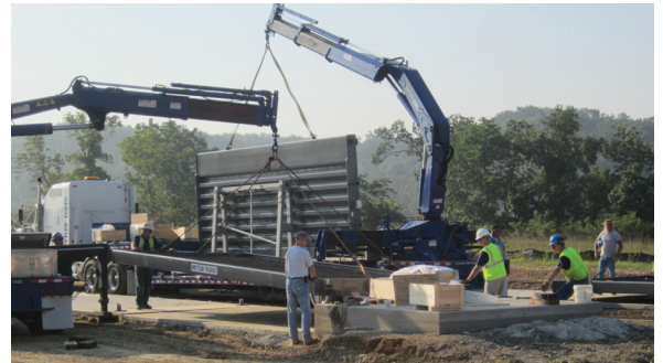
These scale delivery trucks are equipped with on-board cranes used to lift and place the weighbridge modules into the scale foundation
