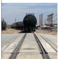
Save money and space with a combination truck/rail scale. A single weighbridge combines a static railroad track scale with a platform for weighing trucks. The rails are recessed to form an even surface that trucks can drive across safely and easily.
