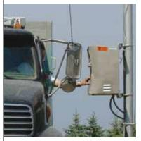
Reduce operating costs with unattended driver terminals. These controllers allow truck drivers to process their own weighing transactions, eliminating the need to maintain a scale house with an operator on duty. You determine what information is collected and how the driver enters it.
