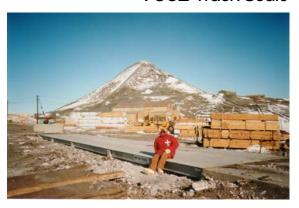
the frozen ground to make room for dynamite sticks. The dynamite was detonated, creating a gap for each footer. The holes were then filled with debris and water, which froze, locking all components into place. The partnership team assembled a technologically advanced weigh solution for extreme weather conditions using the 7562 DigiTOL TRUCKMATE Scale. The scale has now been in service for more than seven years and has been trouble free, even in these extreme conditions.
