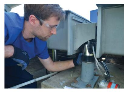
tract the large mechanical components underneath, and replace them with custom-engineered mounts for the 90-ton capacity POWERCELL PDX load cells. By simultaneously replacing the rails on the existing scale deck, the customer would get like-new performance at a fraction of the cost of a new rail scale. This combination of performance and value made the customer's decision to upgrade the rail scale an easy one.
